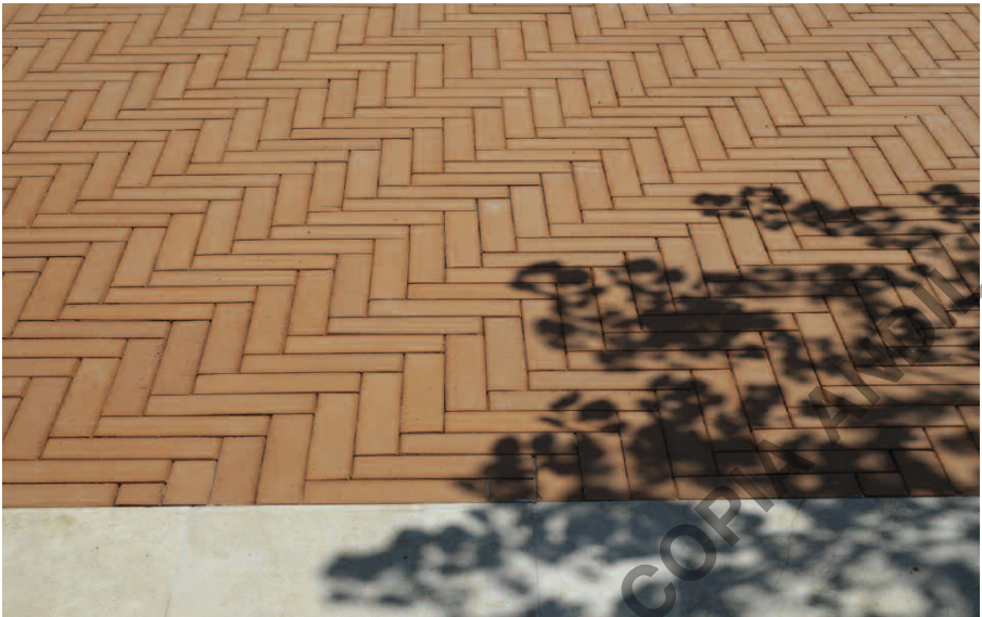
Extruded "sestini" floor with siloxanes in aqueous solution based water-repellent protection.
