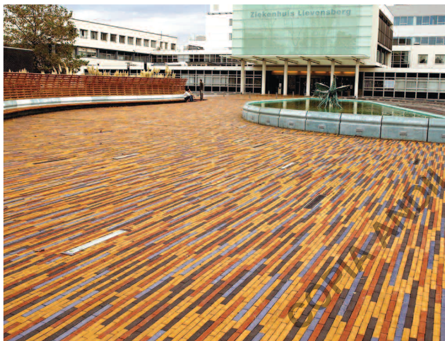
N. Korteweg e N. Zimmerman. Clay paving of the entrance to the Bergen op Zoom (NL) hospital.
