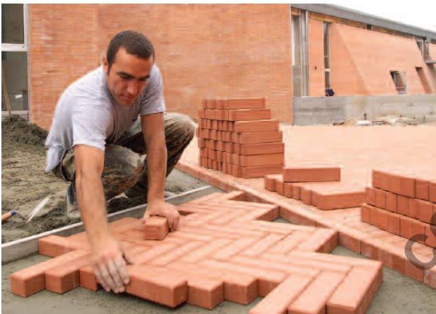
Floor with "sestini" laid with "dusting" technique.
