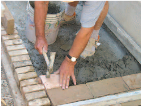
“Masonry” laying technique.
